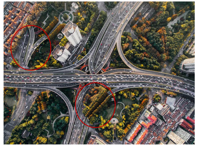
Fig. 14. Incorrect patch locations can lead to implausible results. In this example, the forest cut off the overpass.
